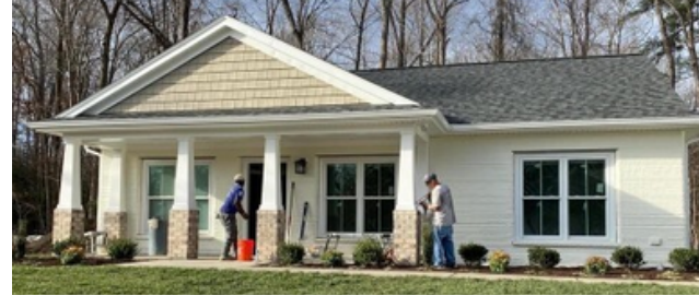
3D printed house by sub-contractor Alquist 3D
